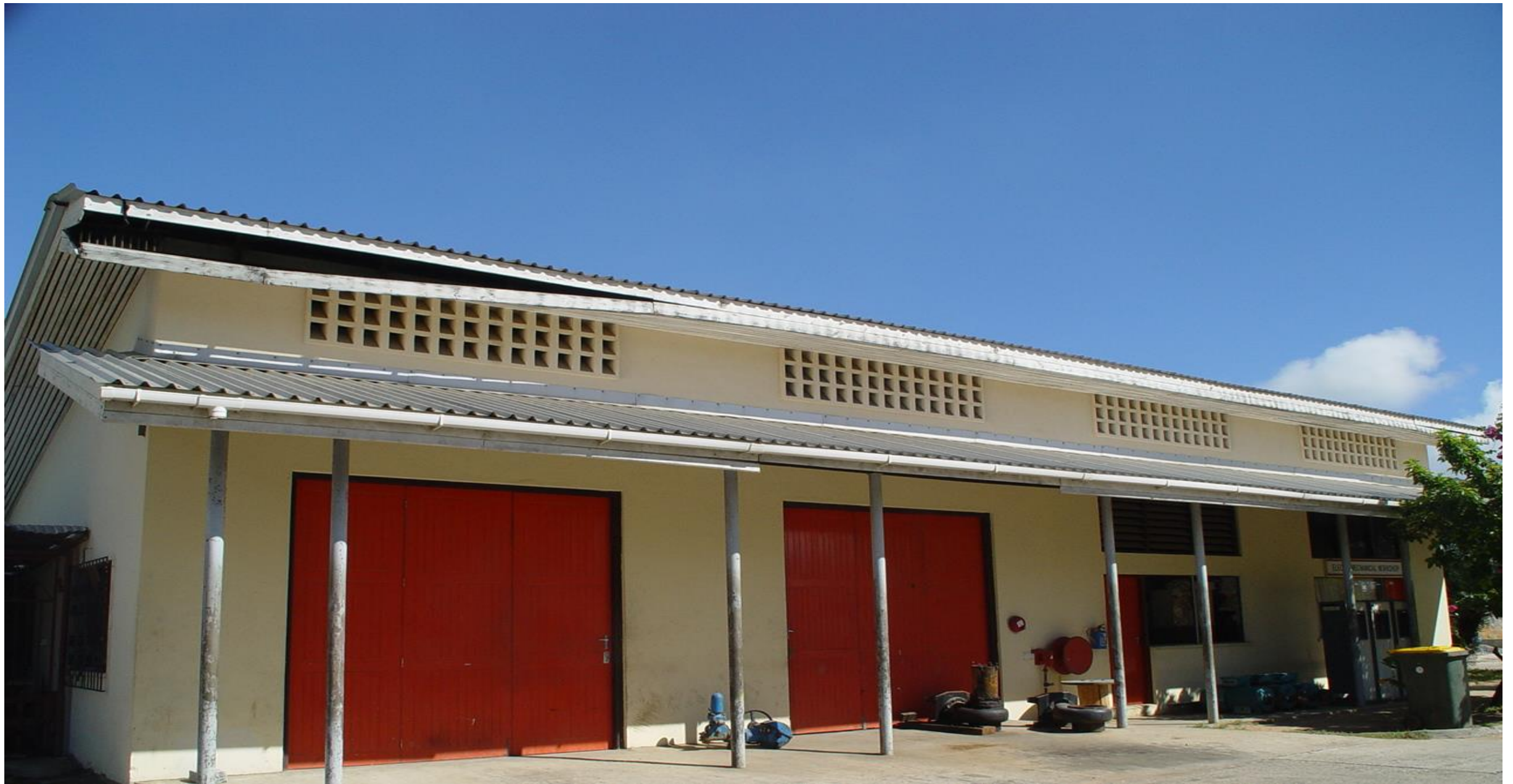
GREATER VICTORIA SEWERAGE AT MAHE
