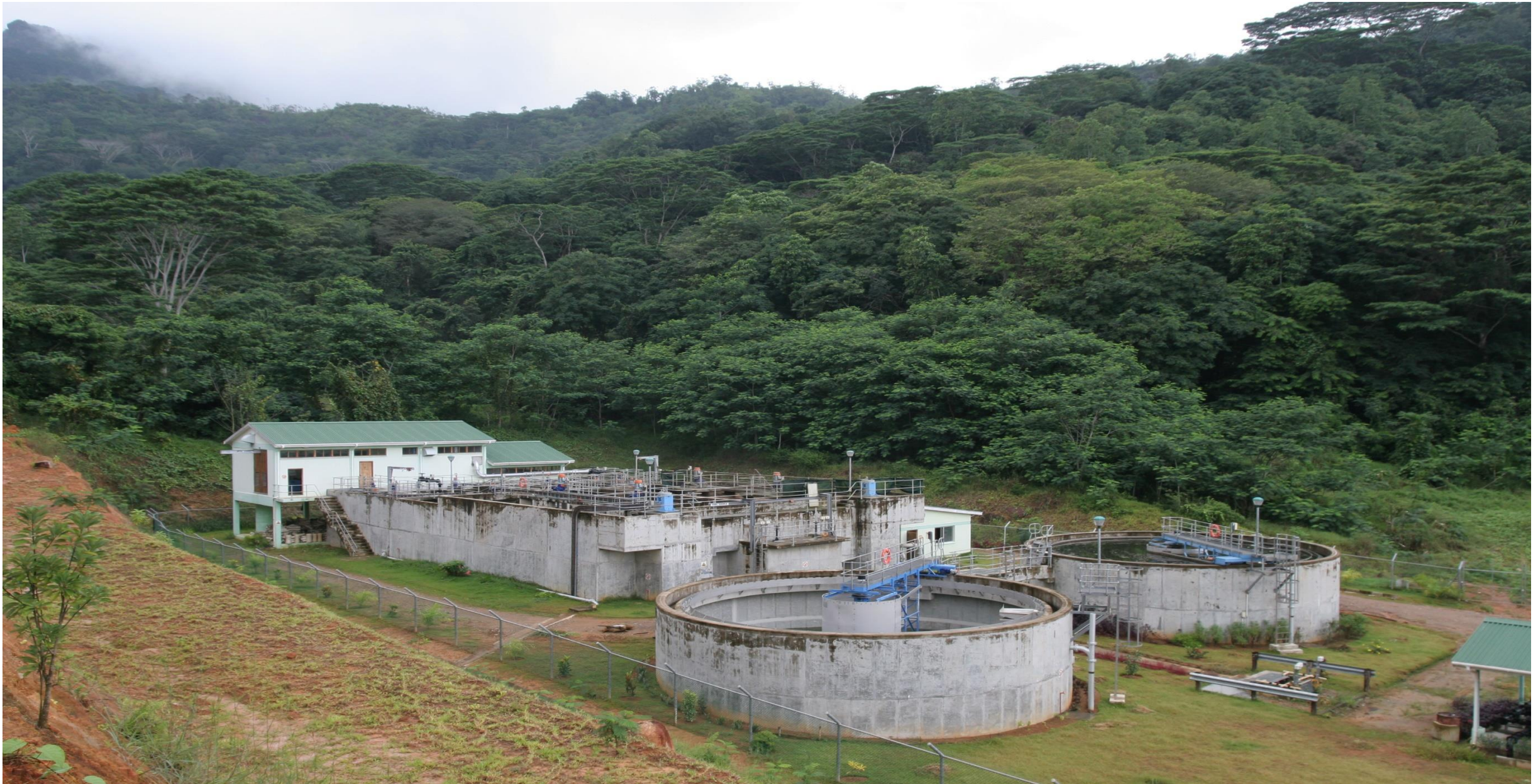
SEWERAGE TREATMENT AT BEAU VALLON MAHE
