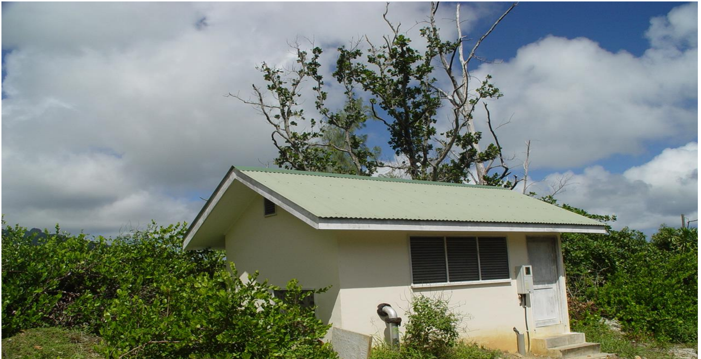
WATER SUPPLY PROJECT AT BARBARAON
