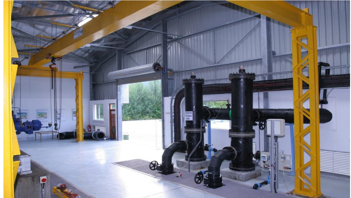
DESALINATION PROJECT WEST COAST AT MAHE
