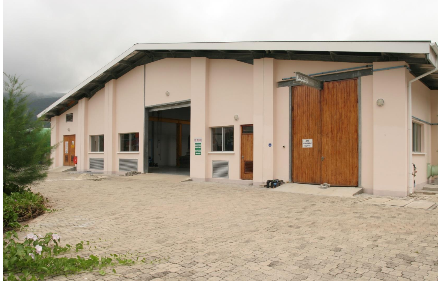
DESALINATION PROJECT WEST COAST AT MAHE
